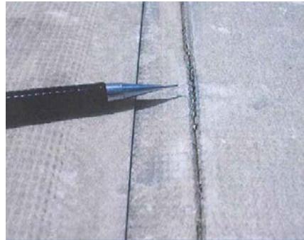
Figure 6: Aged TPO Membrane Problems
